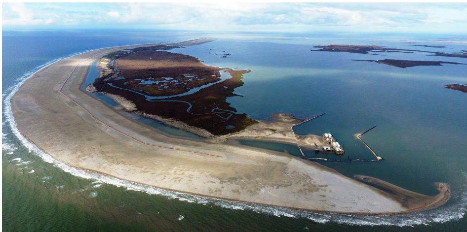
OCS sand was used to restore the Caillou Lake Headland in offshore Louisiana. Photo credit: Great Lakes Dredge and Dock
