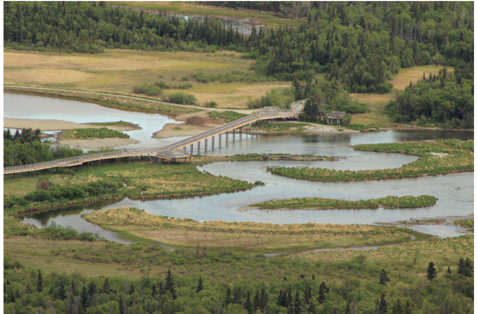
Bird’s-eye view of bridge span, elevated walkways, and three large and two small viewing platforms. Photo credit: R. Jensen, NPS
