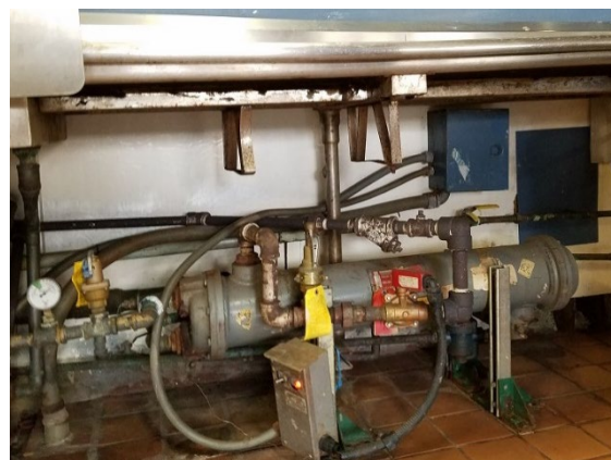
Utility services to base of a dental chair and starter sitting on floor in kitchen
