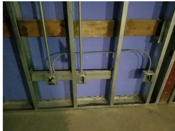
Metal-clad cable used extensively in ongoing project, not allowed by DoD or VA criteria
