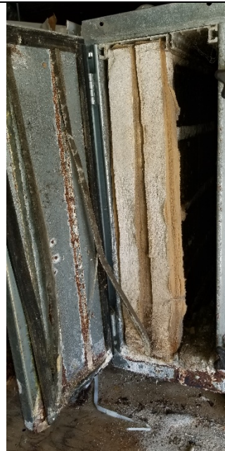
Outside Air Filters
