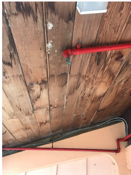
Typical Roof Construction with Sprinkler
