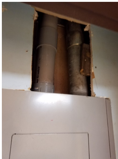
Typical open equipment with exposed wiring and use of PVC conduit indoors
