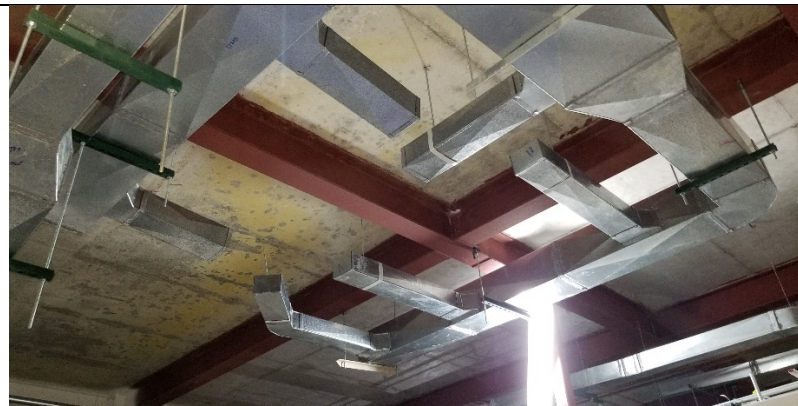
Duct rough in above the Operating Rooms for Laminar Flow Diffusers.
