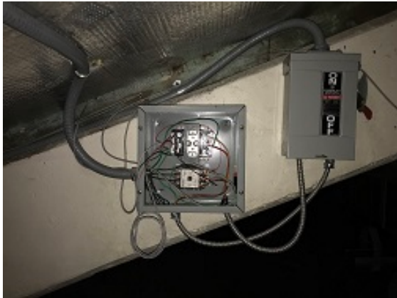
Typical open equipment with exposed wiring
