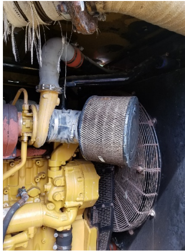
Temporary Diesel Generator that Supports the New System, Showing Effects of the Elements
