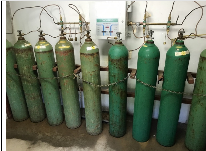
Functional Oxygen Manifold
