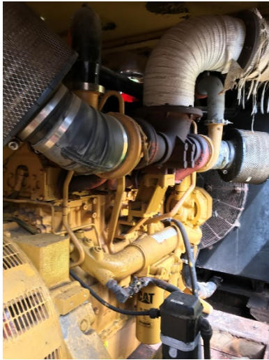
Temporary Diesel Generator that Supports the New System, Showing Effects of the Elements
