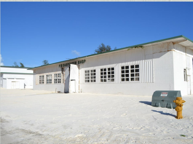
Clean fill around the Carpenter Shop
