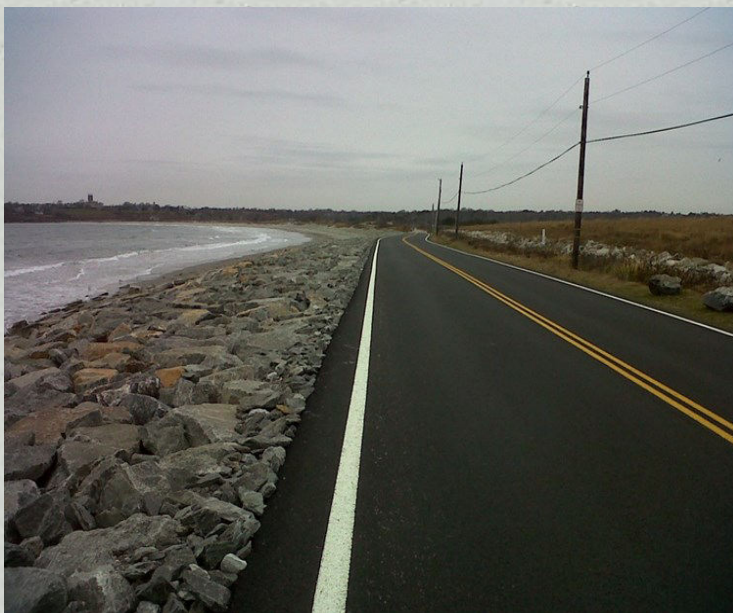
Road that was replaced after Hurricane Sandy. Landfill is on the right side of the photo adjacent to the road
