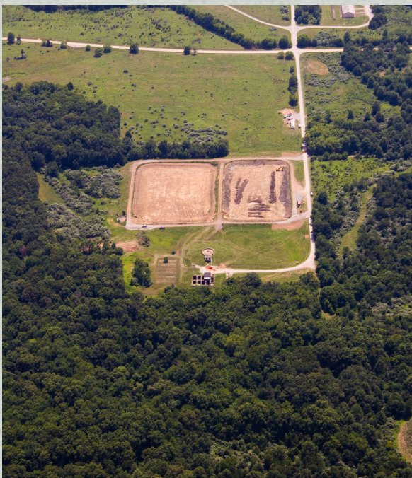
The former wastewater treatment plant that received contaminated industrial wastes before cleanup
