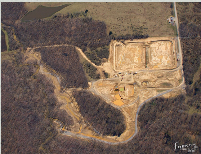
The former wastewater treatment plant after remediation
