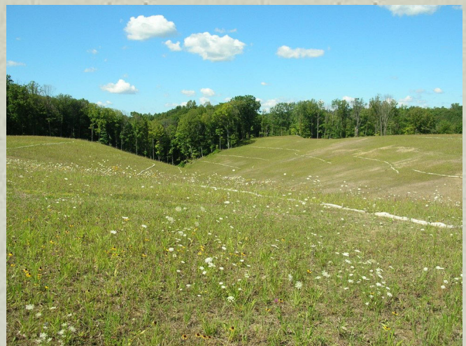
After completion of contaminant excavation and initial re-vegetation of the Site
