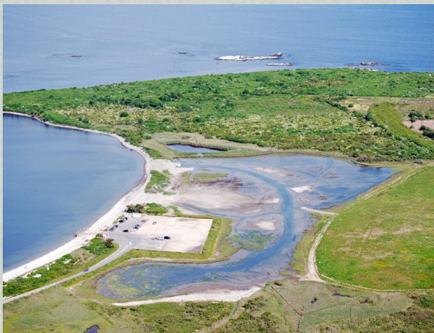
Landfill after remediation
