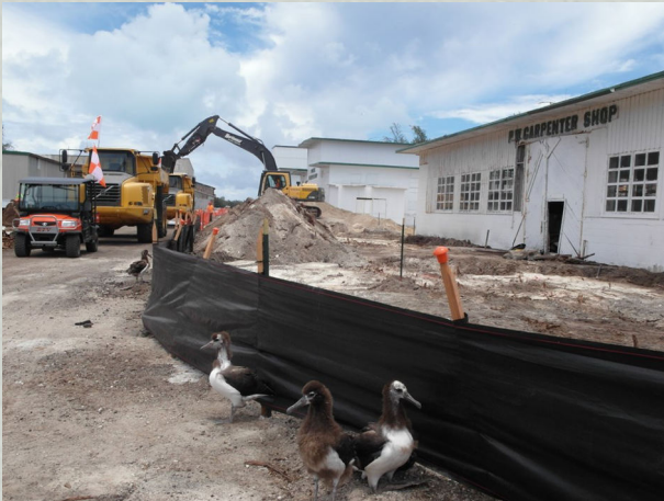
Excavation of contaminated soil around the Carpenter Shop
