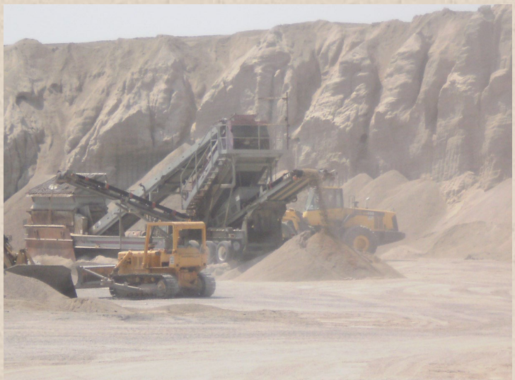
Chat removal activities at Tar Creek
