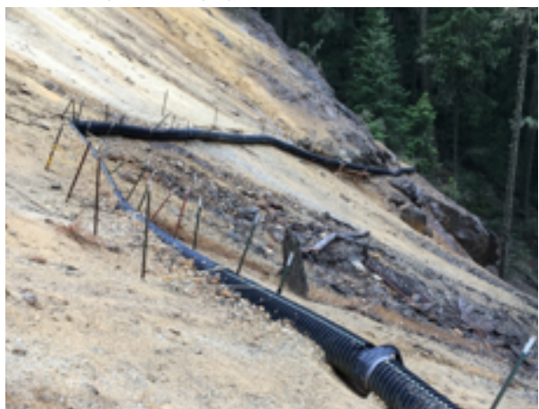
Acid mine drainage diversion system scheduled for replacement in 2019 by BLM to protect watershed water quality. (Photo: John Barber, BLM)
