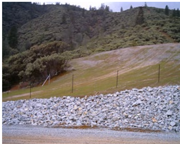
Before and after photos of the excavation, consolidation, and capping of pyrite contaminated soils at the Matheson Ore Transfer Station, near Redding, CA.
