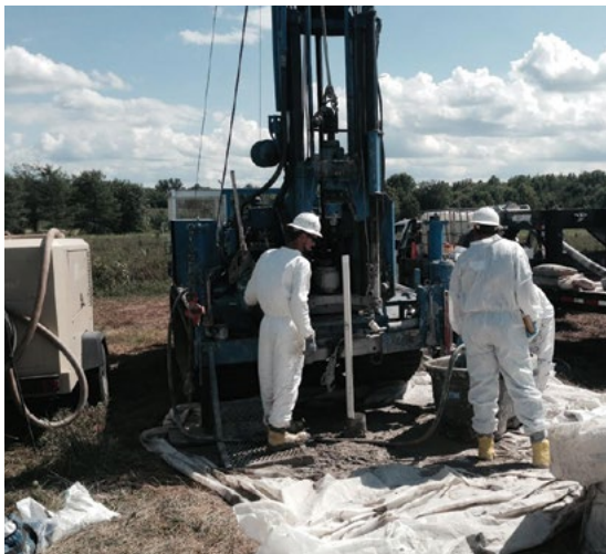
Groundwater monitoring well installation at the Crab Orchard facility. (Photo: FWS)
