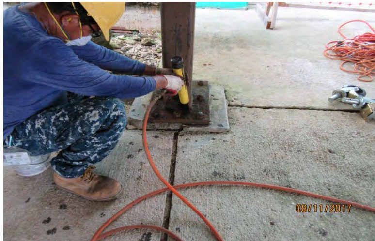
Figure 36 – Column repair at GDOE's Southern High School
