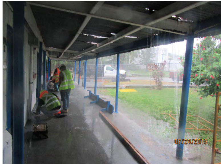
Figure 35 - GDOE covered walkway repair
