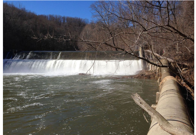
The Bloede Dam on the Patapsco River in Maryland before it was removed in 2018. Photo credit: Rick Bennett, USFWS
