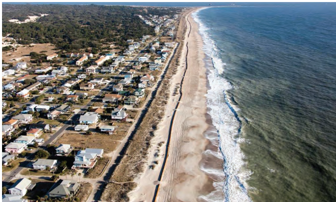
The U.S. Army Corps of Engineers restores the coastline of St. Augustine Beach, FL, for protection and recreational use. Photo credit: Mark Bias, USACE
