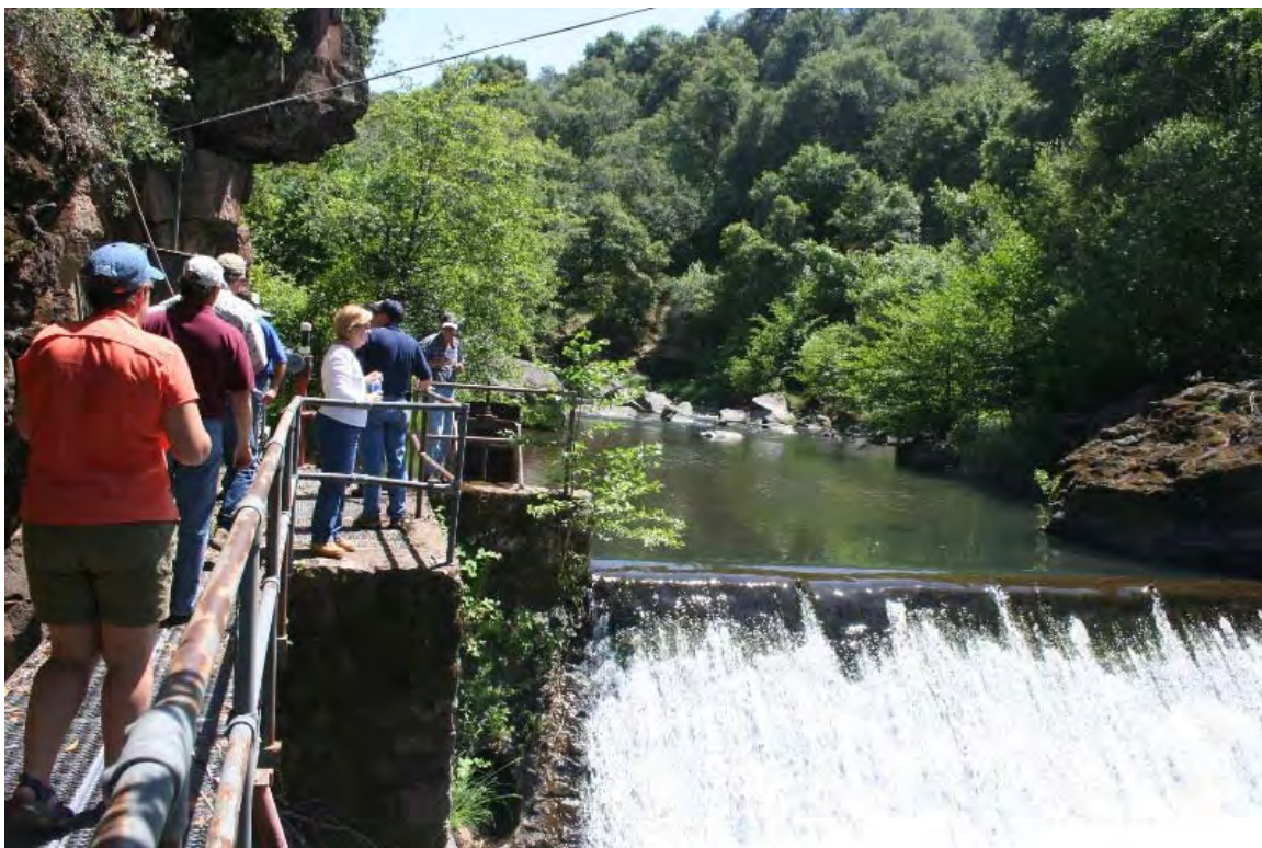
Wildcat Dam to be removed in project to restore fish passage for Chinook salmon and steelhead on the North Fork of Battle Creek
