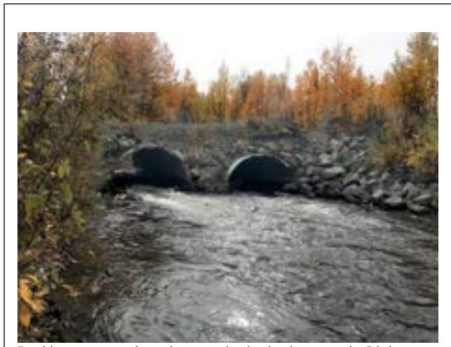
Looking upstream through two undersized culverts on the Little Tonsina River in Alaska. Photo Credit: USFWS
