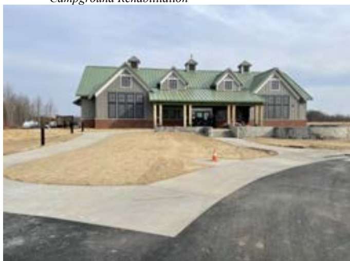
Figure 2. Bombay Hook NWR – Replacement Multipurpose Building Under Construction
