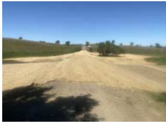
The levee and culvert after repairs.
