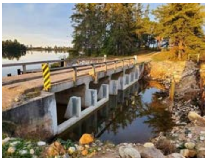
Figure 3: Seney NWR – Replacement Auto Tour Route Bridge
