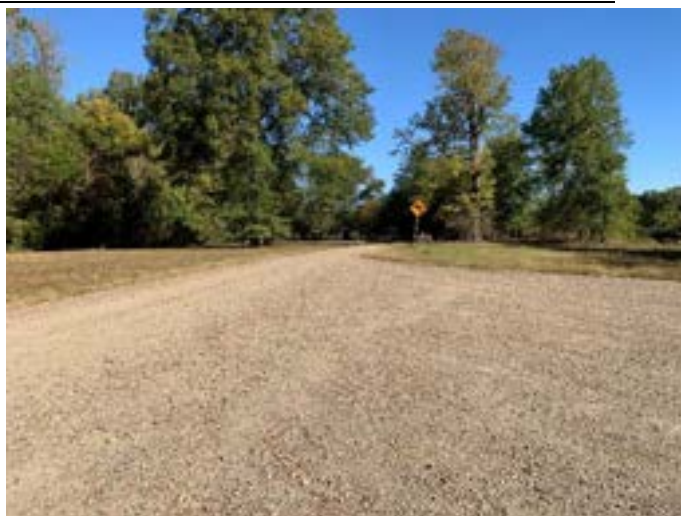
Figure 1. Dale Bumpers White River NWR – Example of Roadway Campground Rehabilitation
