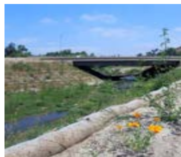
Undercrossing to facilitate wildlife crossing. Photo by USFWS
