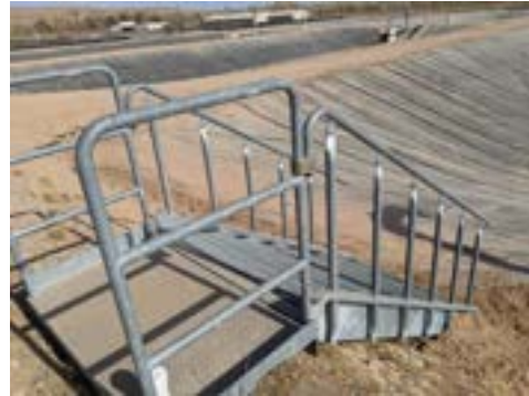
Newly lined ponds and access stairs
