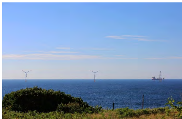
Block Island Wind Farm Project
