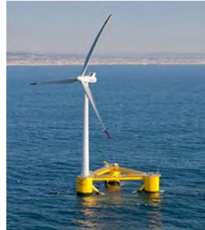
A full-scale prototype of the WindFloat device
