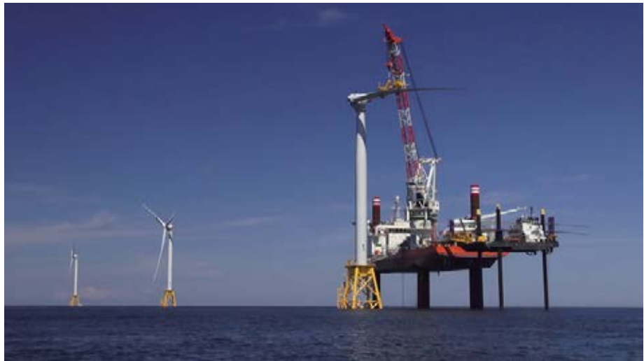
Installation activities at the Block Island Wind Farm, RI.
