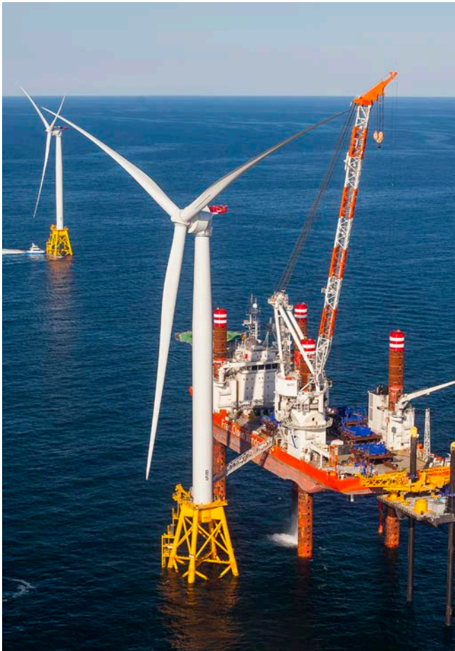
Block Island Wind Farm, New Shoreham, RI.
