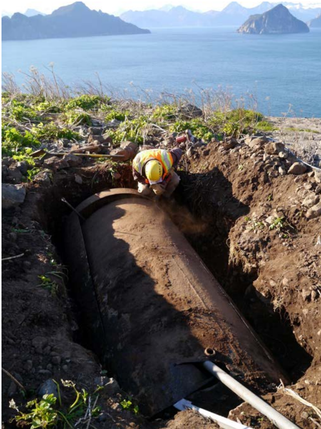
Removal of an underground storage tank on Barwell Island in the Alaska Maritime NWR, AK.
