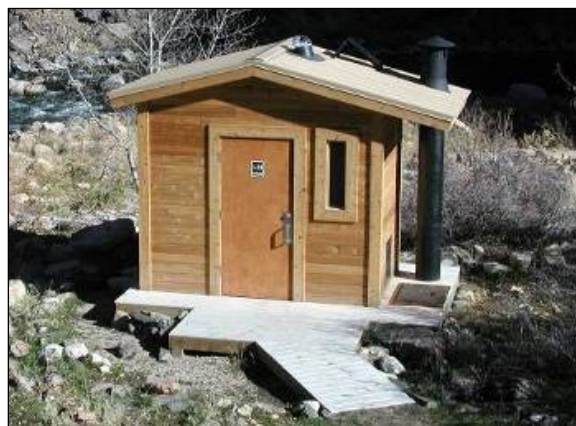
New vault toilet for public use at Gunnison Gorge
