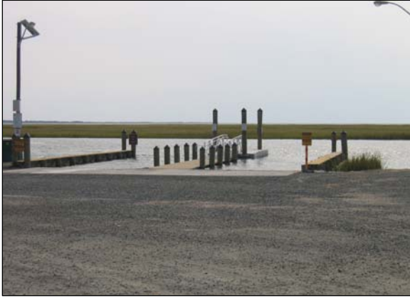
Refurbished boat ramp features solar lighting
