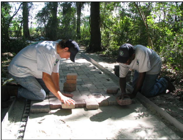
YCC workers improving a walkway
